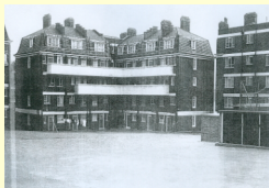
Before - Courtyard (1930's)
